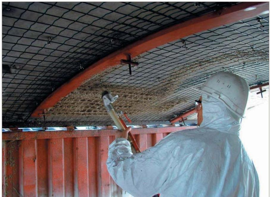
Fig. 9. A 47 mm thick Firebarrier 135 lining being sprayed onto plastic-coated wire mesh fixed to the tunnel segments—in a 1350°C fire this keeps the temperature of the segments under 200°C for at least two hours
