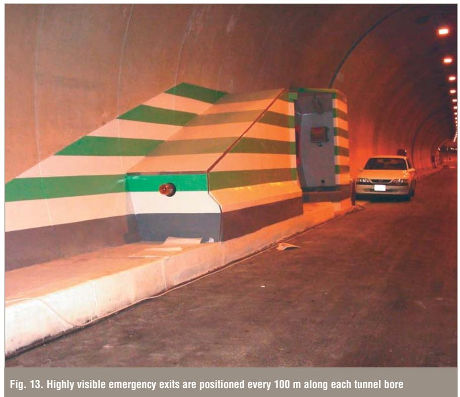
Fig. 13. Highly visible emergency exits are positioned every 100 m along each tunnel bore
