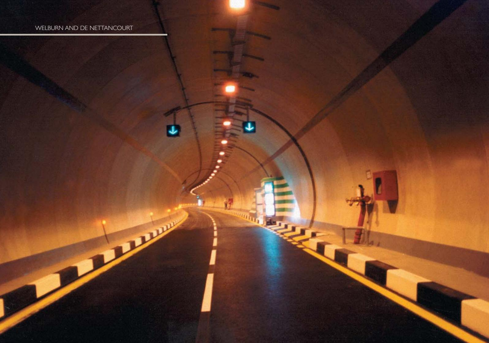
Fig. 10. Completed lining has colour variations and suffers from micro cracking, but this does not affect fire properties
