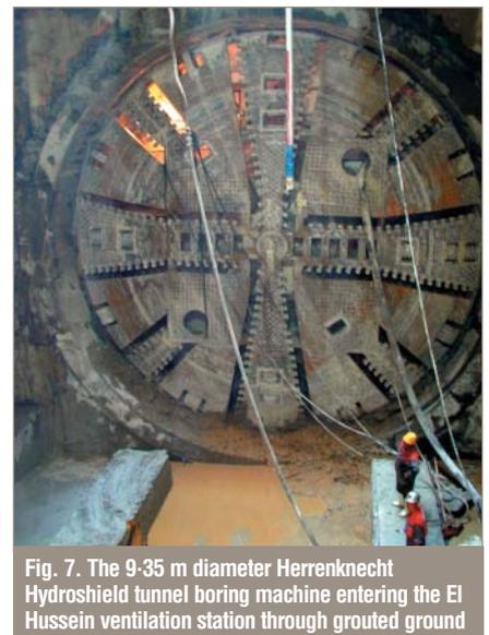
Fig. 7. The 9.35 m diameter Herrenknecht Hydroshield tunnel boring machine entering the El Hussein ventilation station through grouted ground
