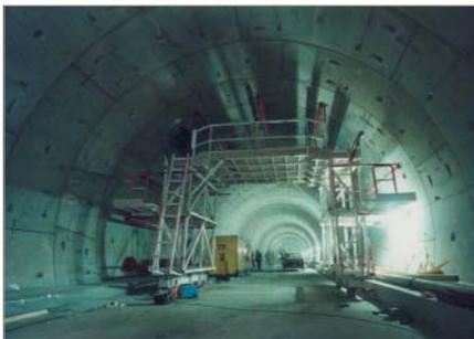
Fig. 8. Tunnel segments are under up to 30 m of groundwater, so it was critical to protect them from spalling damage during a fire
