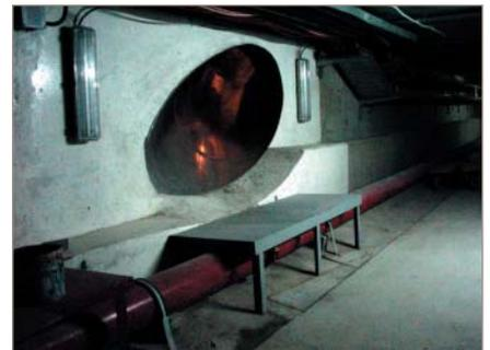
Fig. 15. Exit from escape chute in technical gallery beneath road deck—positive air pressure prevents smoke entering
